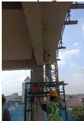
Gambar 7 Proses Pengelotan Mullion
