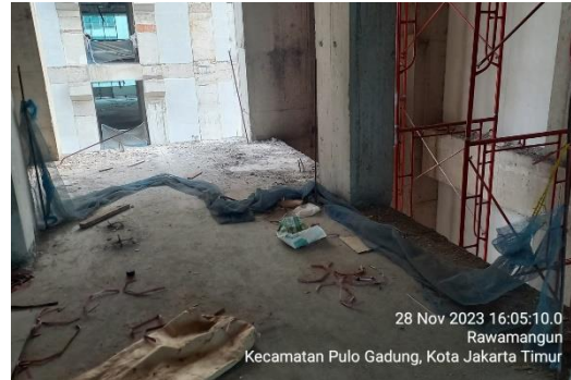
Gambar 2. Void area Lift Passenger Lantai 5 Proyek UNJ
