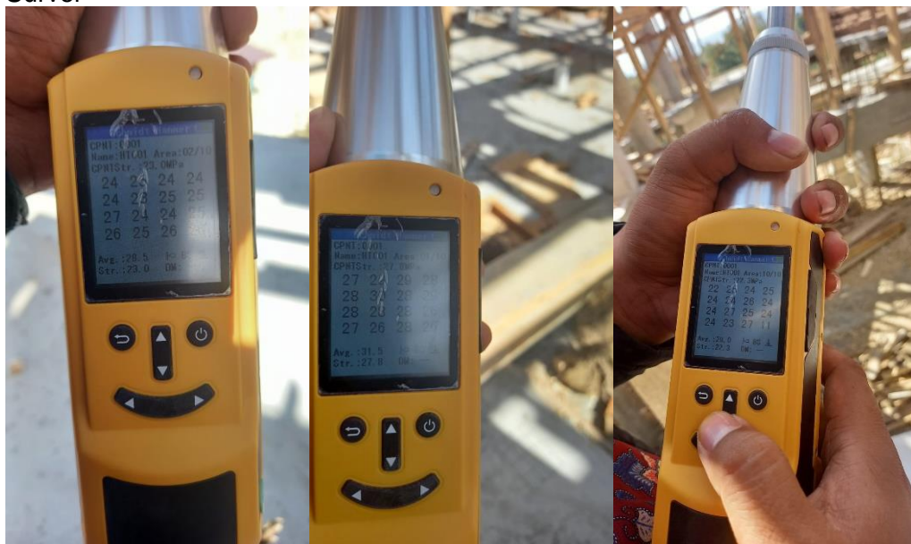
Gambar 4. Data Uji Hammer Test 1
