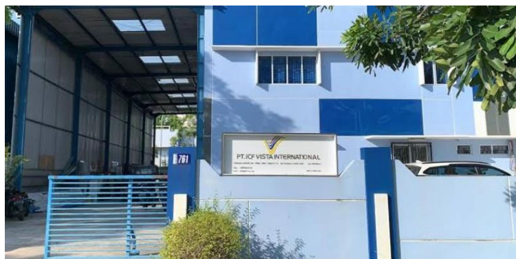
Picture 1.2 PT. ICF Vista International Source: PT. ICF Vista International (2020).
